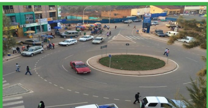
Kitabi-Crete & Huye Urban Road in Rwanda where the contractor’s works met the client’s expectations
